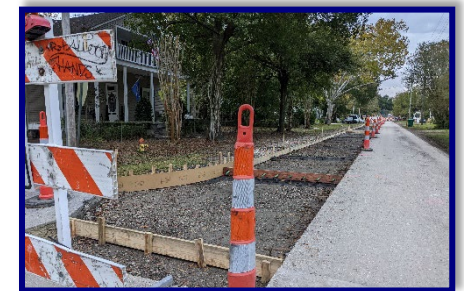
Carey Street Pavement Reconstruction
